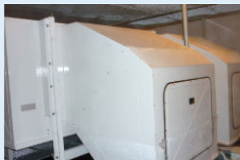
The evaporators are provided with service hatches for easy access to the fans
