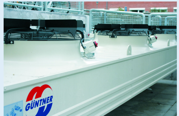
S-GVH gas cooler condenser with fans wired in pairs to the repair switch
