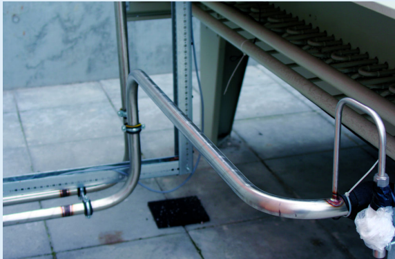
Gas cooler condenser in stainless steel
