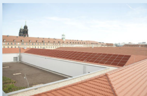
View of the roof after installing the sight screen
