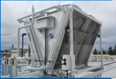
▲ The spraying of the Güntner V-SHAPE Vario, type GFD, automatically activates at an ambient temperature of 27 °C and thus allows for cooling the ethylene glycol down to a lower temperature level than that of the ambient temperature.
