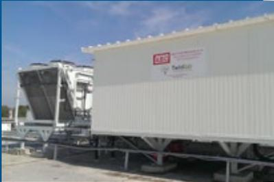
▲ The enclosure for the additional decentralised central cooling facility and the condensers needed to be located, for lack of space, on the roof exactly above the production.
