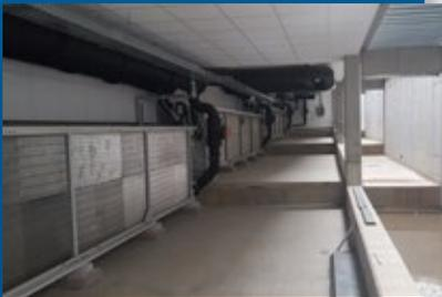
▲ Altogether seven Güntner VERTICAL Vario GFV units with a total cooling capacity of 1,400 kW provide need-based refrigeration of the different rooms of the castle.
