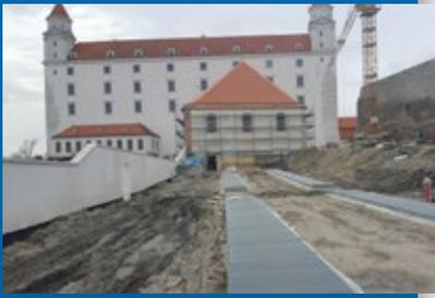
▲ The entire supply engineering of the castle was installed below ground level for optical reasons. The ambient air for the Güntner fluid coolers is taken in via one duct before the heated air is dissipated through the second duct.
