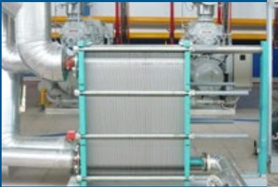
▲ A thermowave plate heat exchanger transfers cold from the central ammonia refrigeration cycle to the water circuit which, in turn, cools the production rooms to an average temperature of 15 °C.
