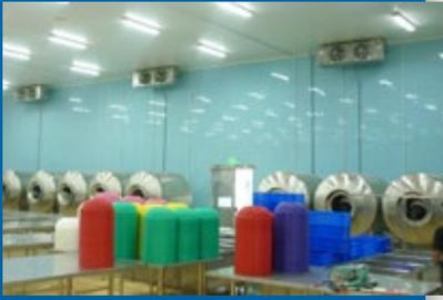
▲ Guntner CUBIC Vario GGHF air coolers ensure a room temperature of 15 °C in the production rooms. As the corrosion potential is very high due to the salt aerosols in the production rooms, Guntner CUBIC Vario GGHF made of stainless steel with AlMg<sub>3</sub> resin-coated fins are used.
