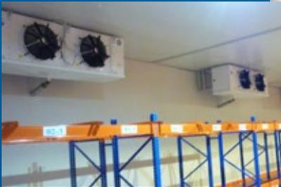
▲ Eight Güntner CUBIC Vario AGHN air coolers and DX evaporators of different sizes evenly distribute cold in the storage rooms.
